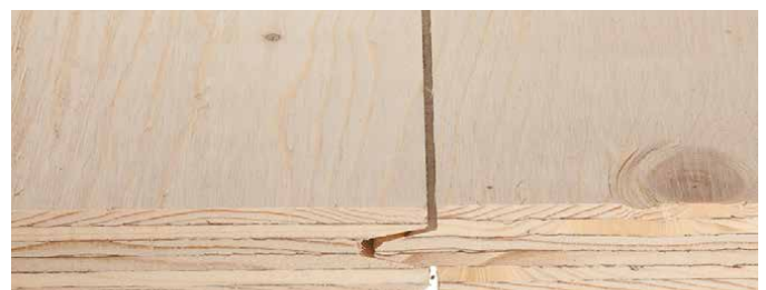
Figure 16. Tongue and groove (TG) joint
