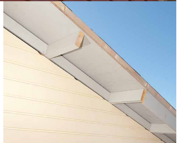
Figure 24. Cantilevers supporting eaves overhang
