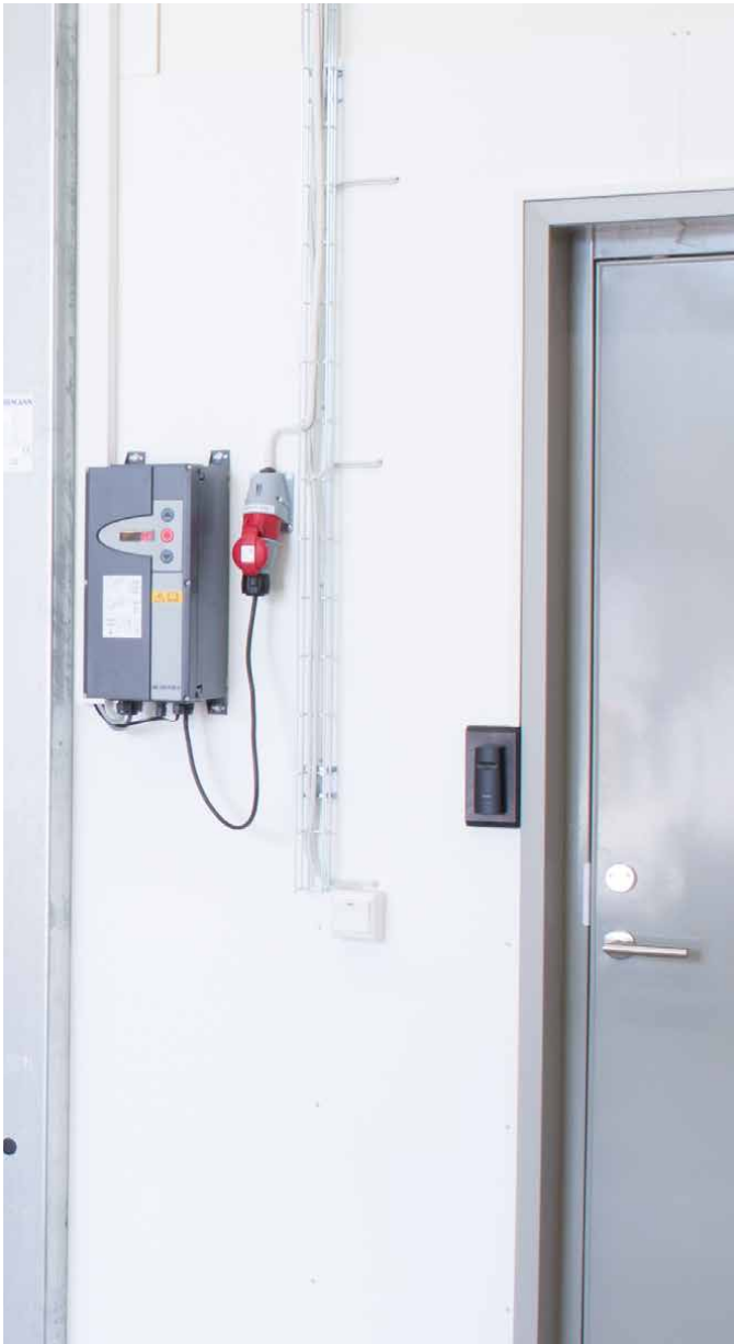
Figure 32. Plywood panel as a fixing base
